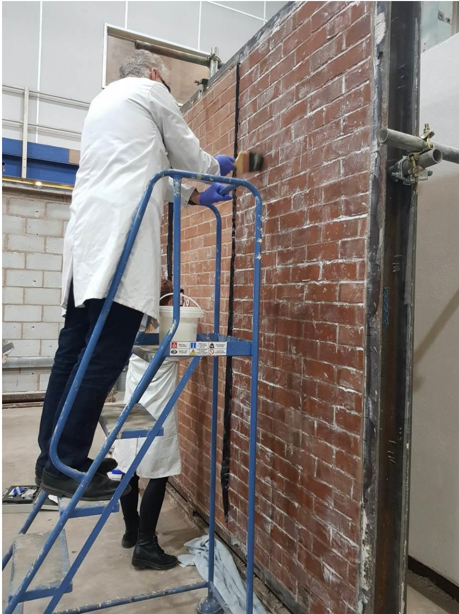
Plate A2-2 – Application of Safeguard Europe Trial Product X116 Masonry Coating
