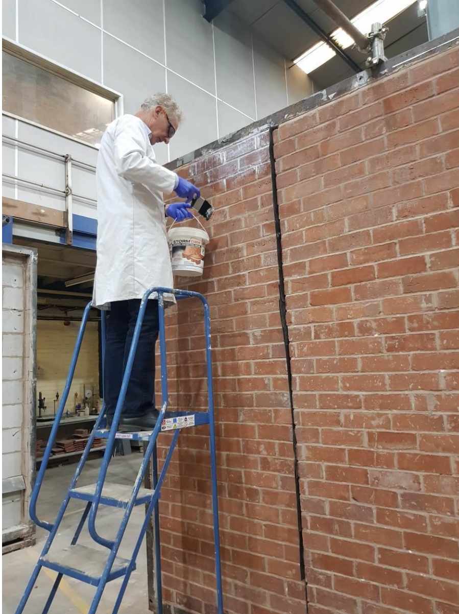
Plate A2-1 – Application of Safeguard Europe STORMDRY Masonry Coating
