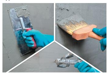
**Drybase®** *TS-PLUS* **Polymer Enhanced Tanking Slurry** can be applied by trowel, brush or suitable spray equipment.
